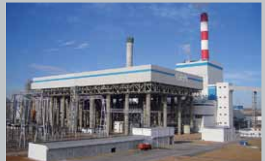
Air Cooled Condenser in a Power Plant in China
