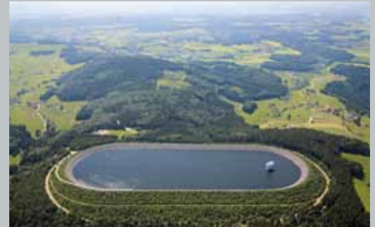
Pump storage plant, Schluchsee, Germany
